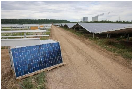
A solar farm is being constructed in Saxony, Germany, using 1.1 million solar modules imported from China (Image: Jan Woitas / Alamy)
